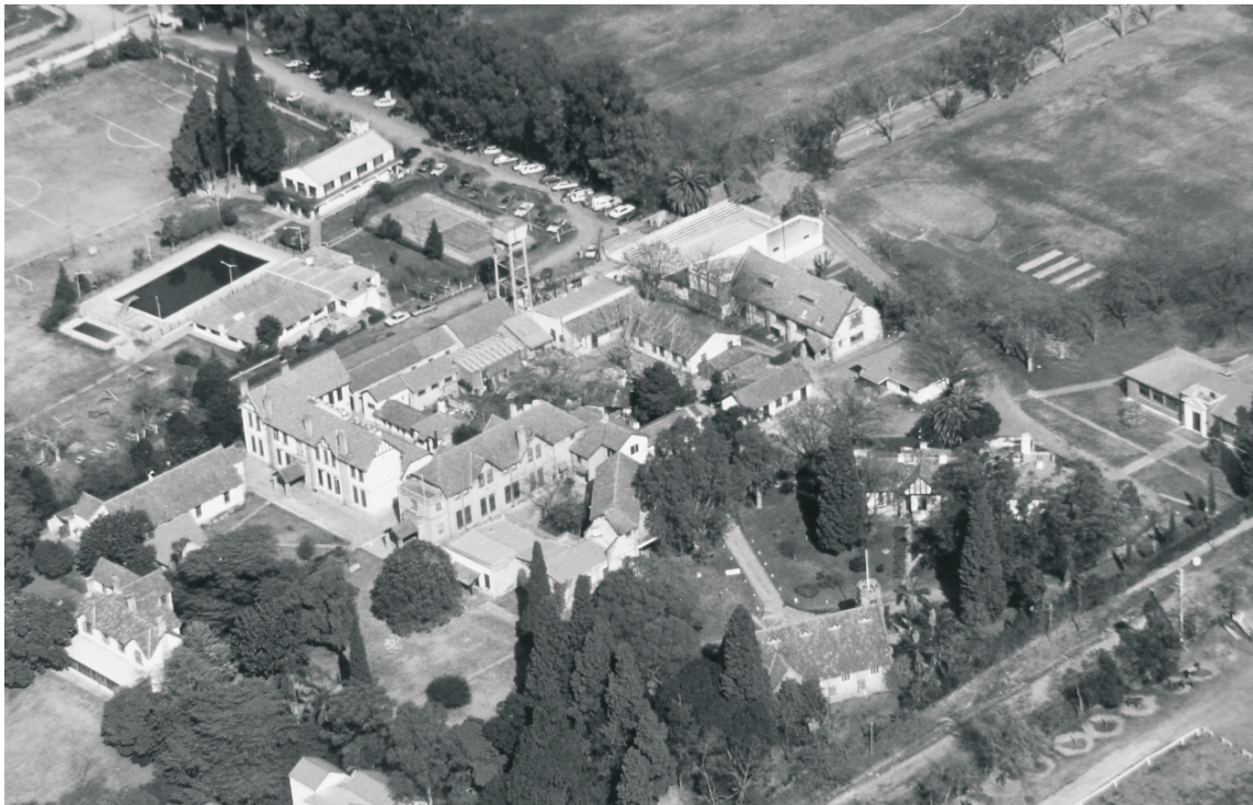
Fig.Nº20: vista aérea, Colegio San Jorge, Quilmes.
