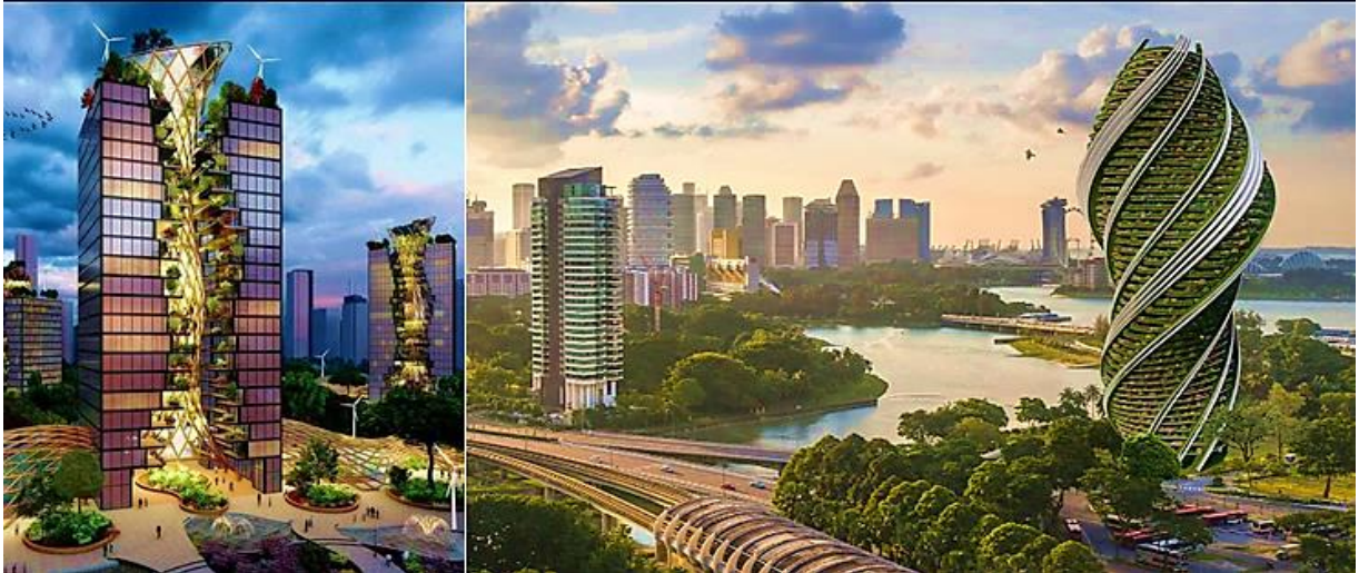
Figura 29 Tree tower Archinature coexisting (Japon) 2022-Helico Sky-Rise.Green Luxury Apartaments (Singapur)-2020
