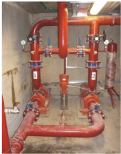
Bomba Jockey Bomba principal Bomba auxiliar
