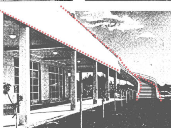
Escalera exterior 50's
