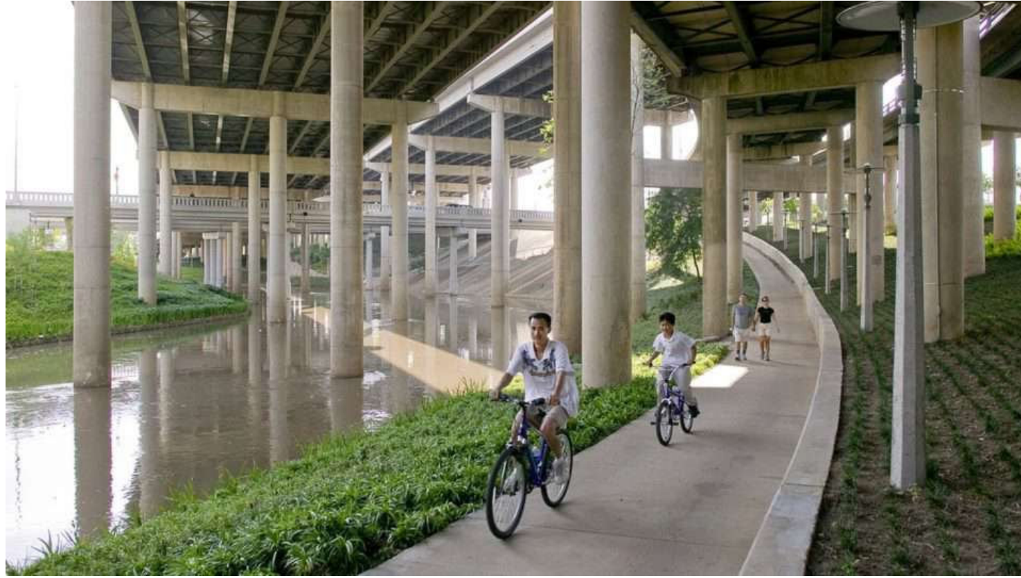
KOGANECHO CENTER Yokohama - 2005
