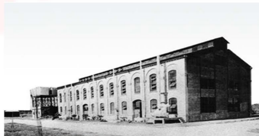
| USINA DEL PUERTO | Ing. Carosio Juan
